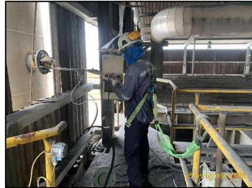
Power Boiler Stack
