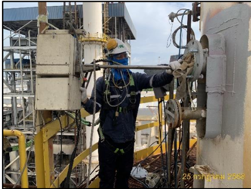
Recovery Boiler Stack
